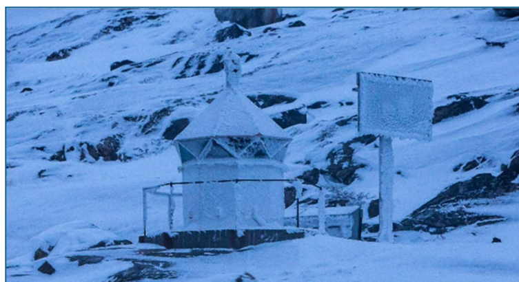
Figure 12 Example of ice on AtoN structure
