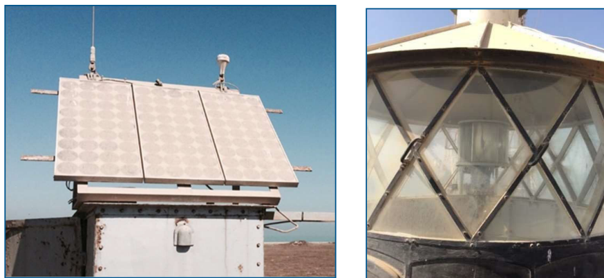
Figure 19 Presence of dust on AtoN device
