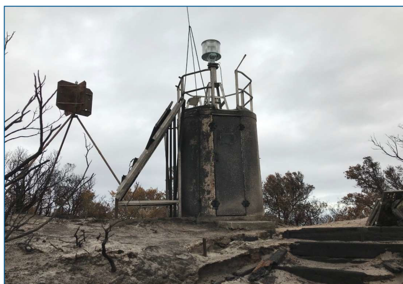
Figure 21 Example of AtoN destroyed by fire
