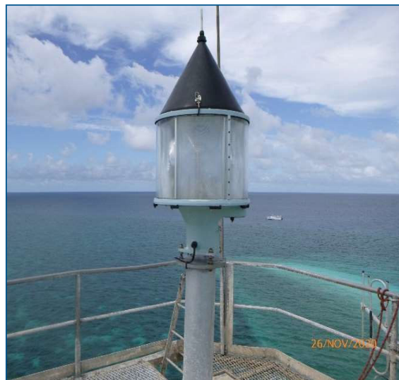
Figure 29 Anti-graffiti product application and Example of AtoN configuration to deter bird roosting
